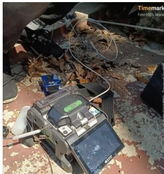
Gambar 7. Splicing core Fiber Optik
